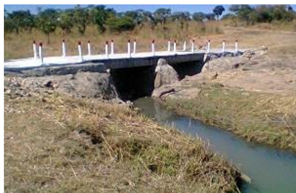
Newly constructed Mwomboshi-Mweemba Bridge
