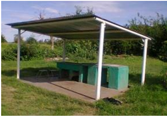
The laundry shelter that was constructed using steel poles. The previous one was on wooden poles.
