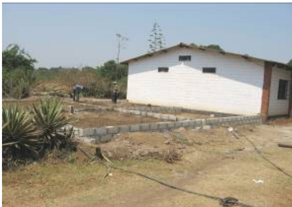
The initial stages of the laboratory construction project
