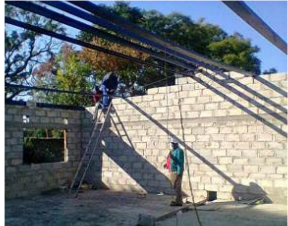
Roof construction being carried out on the Laboratory construction project
