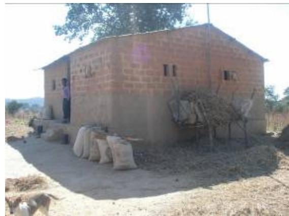
One example modern house being constructed in Kalwelwe Settlement Village
