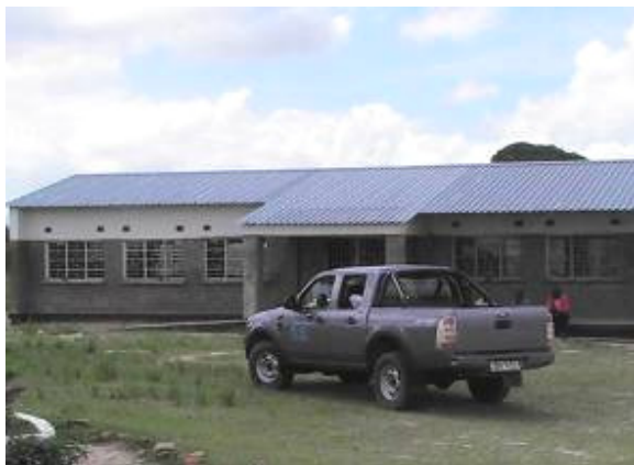
Part of Kalwelwe Primary, built by the Government. It started as a community school
