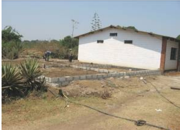
Part of the new laboratory at the initial stages of construction
