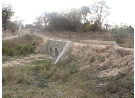
The bridge constructed in 2013
