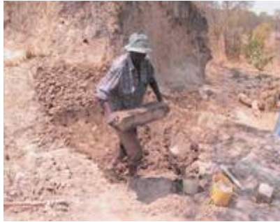
Bricks being moulded from the anthill soil
