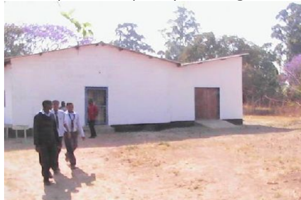
Completed carpentry building
